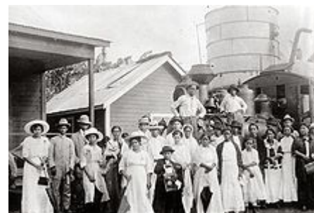
Main Railroad station in La Ceiba, Honduras in 1920.
